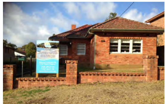
Douglas Street Aged Care Office
